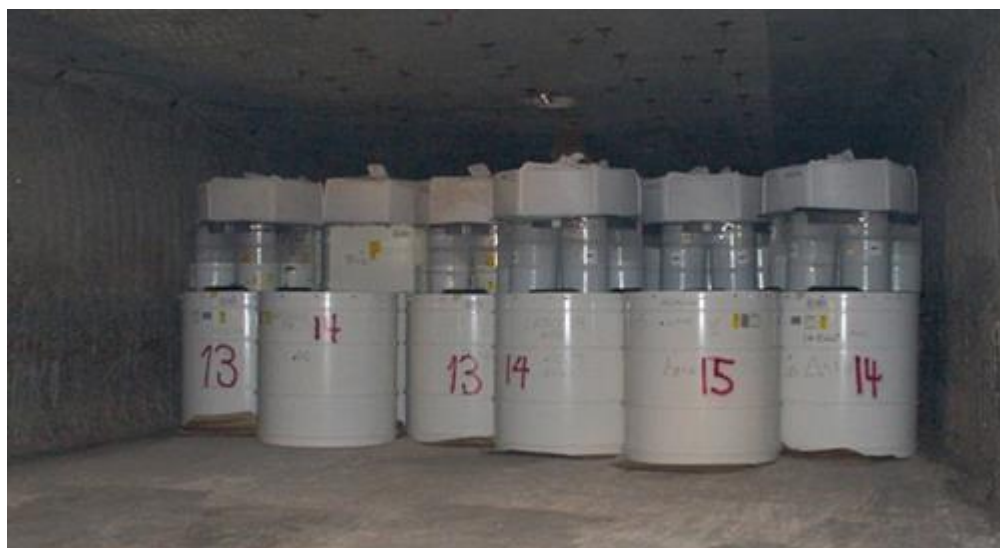
Figure MgO- 1. Supersacks of MgO Emplaced on Top of the Waste Stacks
