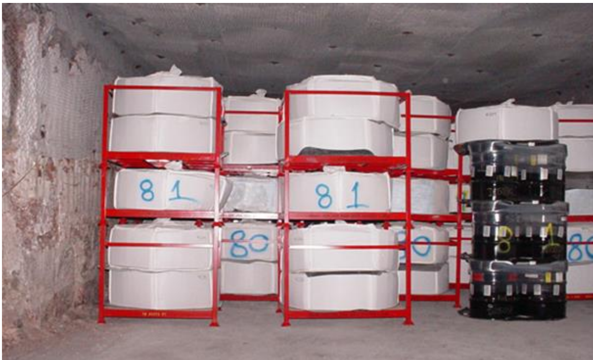
Figure MgO- 2. Racks Used to Emplace Additional MgO
